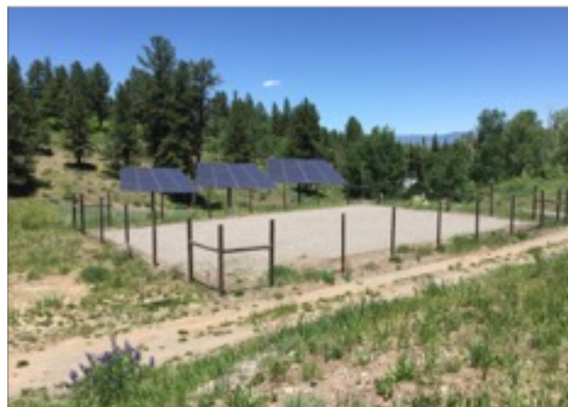
The waste water treatment plant.
